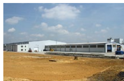
EUROS Polska Sp. z o.o., production facility in Żory-Warszowice, Poland
